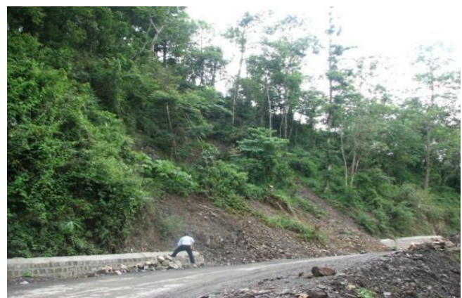
Figure 8. Debris slide in crushed zone
