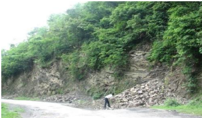
Figure 6. Debris slide in fractured rocks
